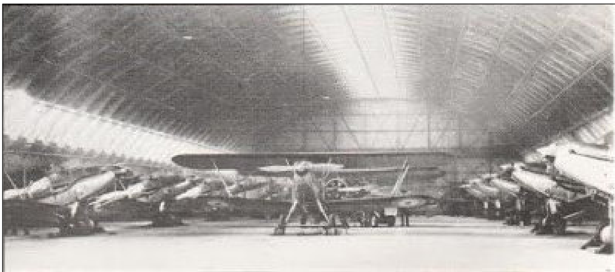
Inside the Lamella hanger
