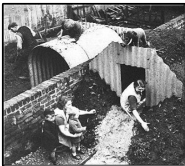
Erecting an Anderson shelter
